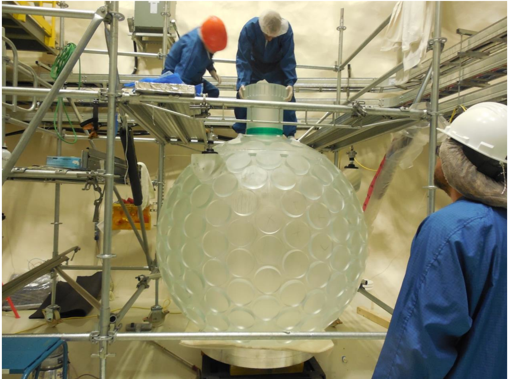
Setup for AV Neck Bond (Reynolds Polymer, Tech. at SNOLAB Jan 2013)
