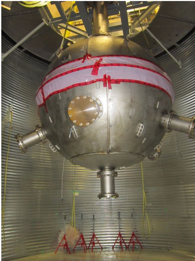
Steel Shell in final installation position, hanging from deck
